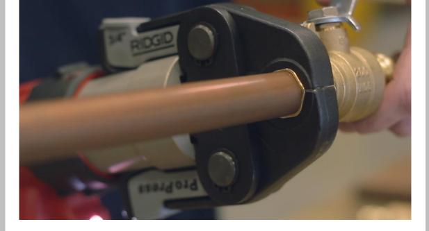
While some joint preparation is required (cutting and deburring), UltraPress valves substantially reduce overall installation time — up to 68%. That's the equivalent of three UltraPress valves installed in the same time period as one soldered valve.
