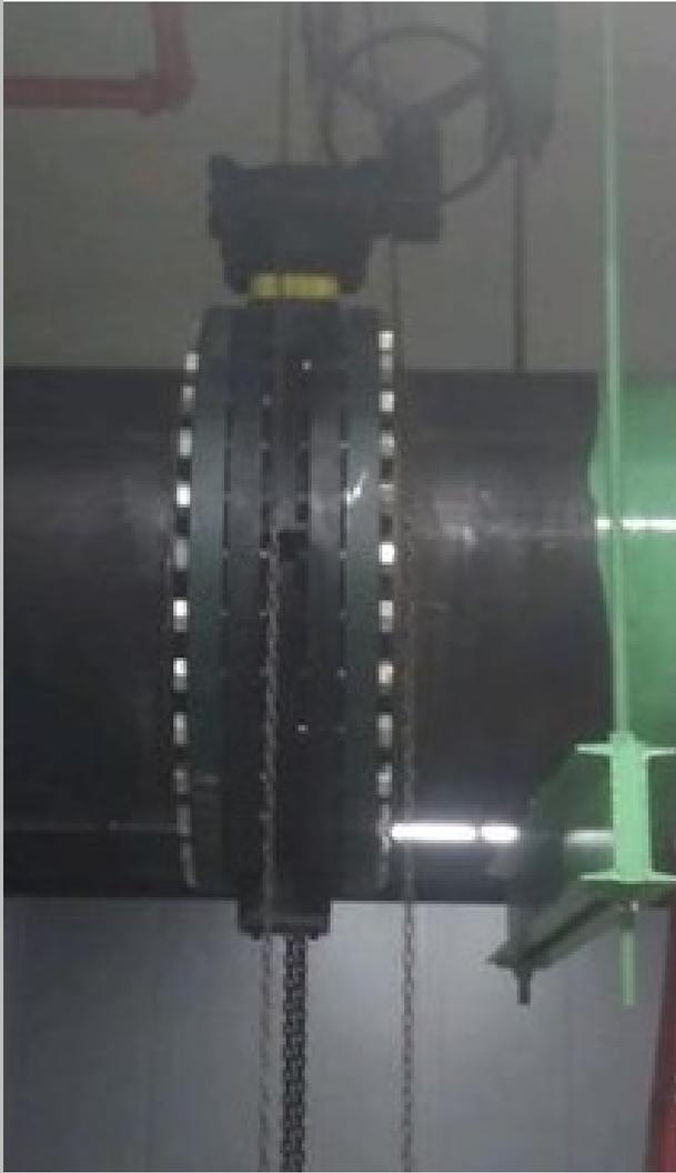
On the other hand, note this installation with a 36" resilient-seated valve. When using such large valves, it's recommended that the stem be installed vertically. Having the valve upright minimizes any side-loading of the bearings and liner, due to the weight of the disc. This is only important in the larger diameter sizes.
