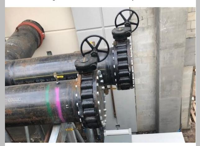
Another note of caution on this topic. Often times butterfly manufacturers rate their valves for standard pressure, but the dead-end capability is de-rated. This is common, even more so on larger, 250 PSIG-rated valves. For instance, on resilient-seated 14" to 24" Milwaukee Valve products that are normally rated to 250 PSIG are derated to 200 PSIG.
