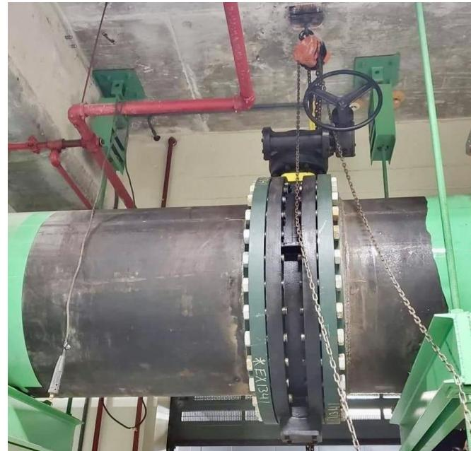
difference between Series A and B, we looked it up. Series B flanges have VERY different dimensions than Series A. They are thinner, utilize more bolt holes, with smaller bolt diameters. Series B can be significantly less expensive but are typically found in non-critical and refurbishment situations. Perhaps someone was trying to save some money by using Series B.
